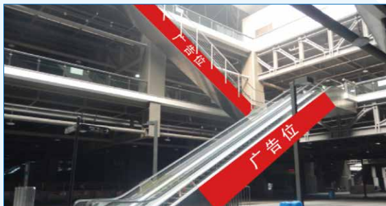
C11 Escalator advertisement - North Skylight
